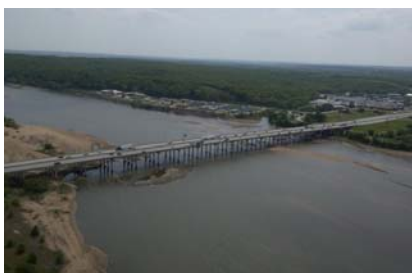
View of the Arkansas River at the I-44 Bridge
