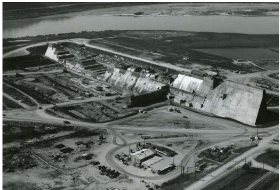
1961 Photograph of Keystone Dam under construction
