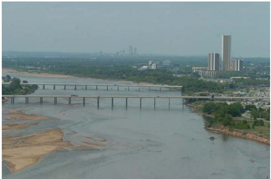
View north along the Arkansas River toward the Creek Turnpike and Jenks Bridges
